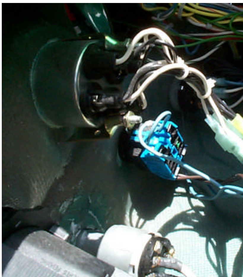
E-Meter, ignition key switch,(bottom), left indicator cluster (top left), direction switch (blue), wiper switch.
